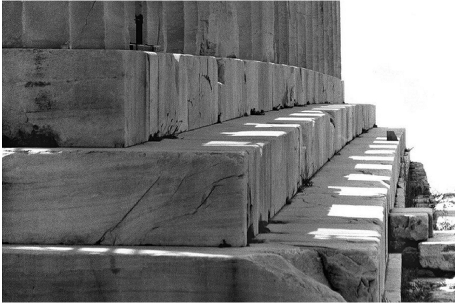
Figure 2. Parthenon, Athens. Photograph by S. Mavrommatis. Optical refinements shown in the upwardly curving base platform, crepidoma , at all three levels.
