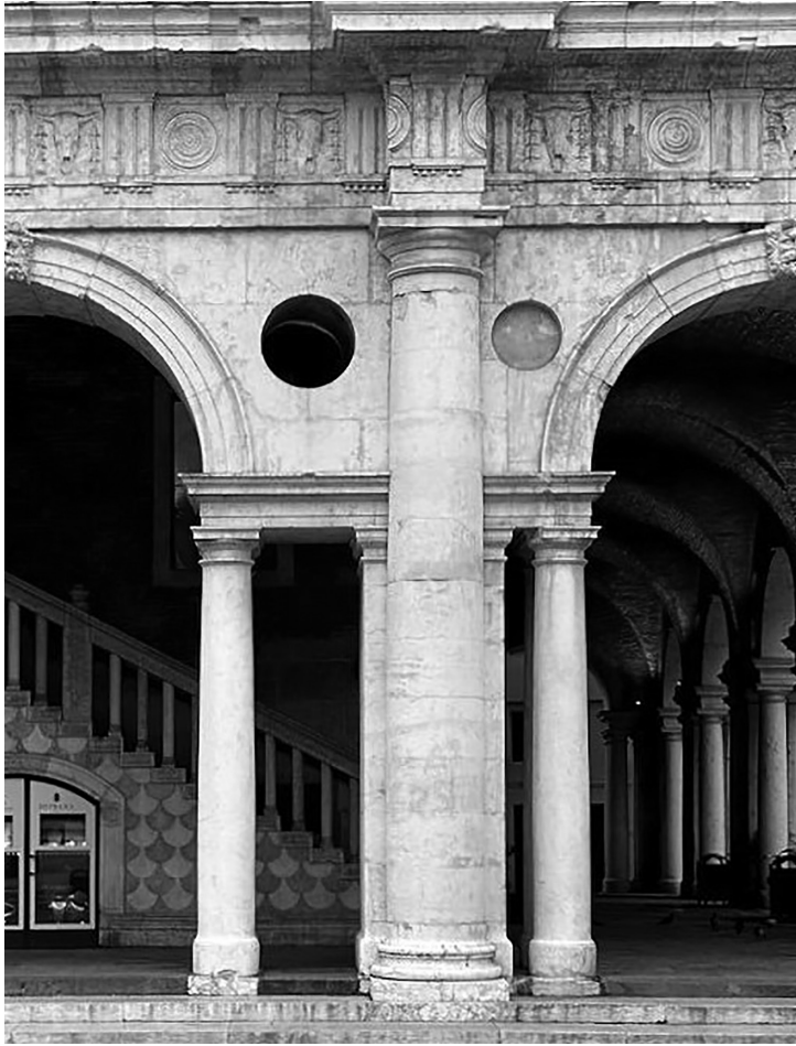
Figure 9. Andrea Palladio, Basilica, Vicenza, 1549, columns, arches, and spacing on front façade. Photograph by D. Leatherbarrow.
