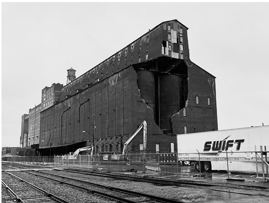
Figure 3. The Great Northern grain elevator. Photograph taken by C. Korsmeyer, December 2021. The interior silos can be seen through the hole caused by wind damage.
